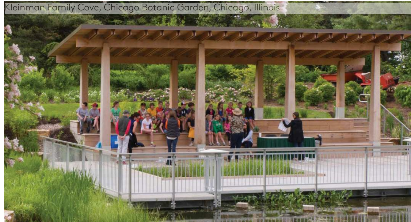
Open air linear pavilion with bleacher seating provides shade without creating a large covered space that can be dark in the center, program storage below the seating
