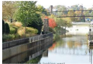
Riverfront Canal Walk looking west
