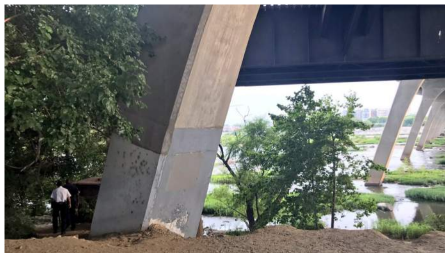
Manchester Bridge support and southern view to the river
