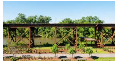
Section of the railway viaduct along the Lowline
