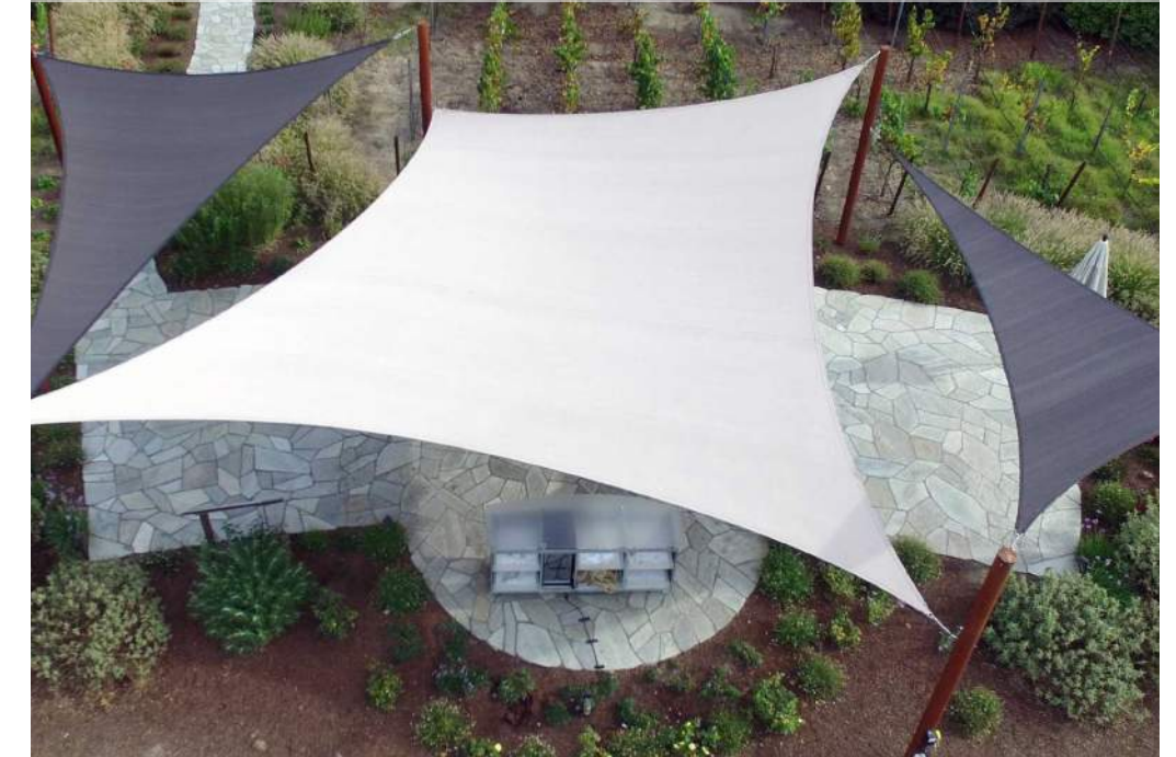
Tensile fabric structures would be used to provide shade over the Central Stair
