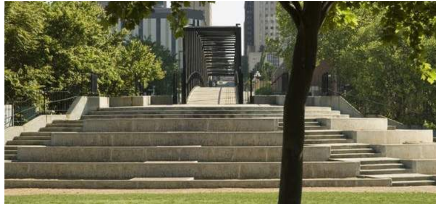
Concrete terraces looking north towards pedestrian bridge
