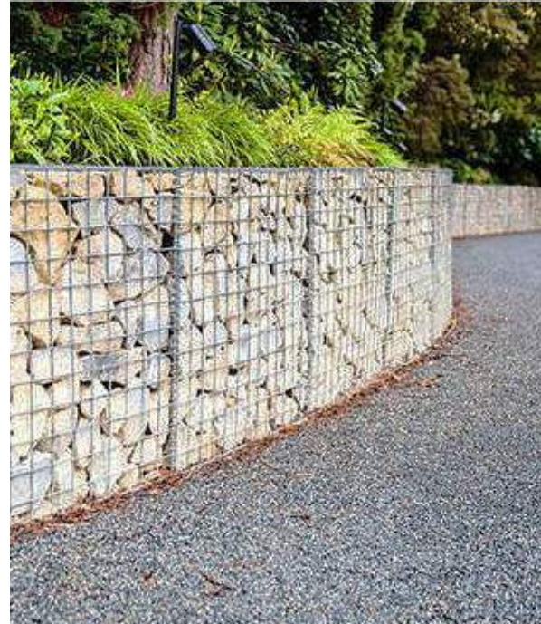
Gabion retaining wall with riverrock fill
