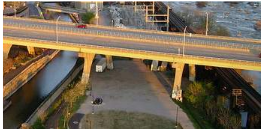
Aerial view of Back Porch area, substation in background
